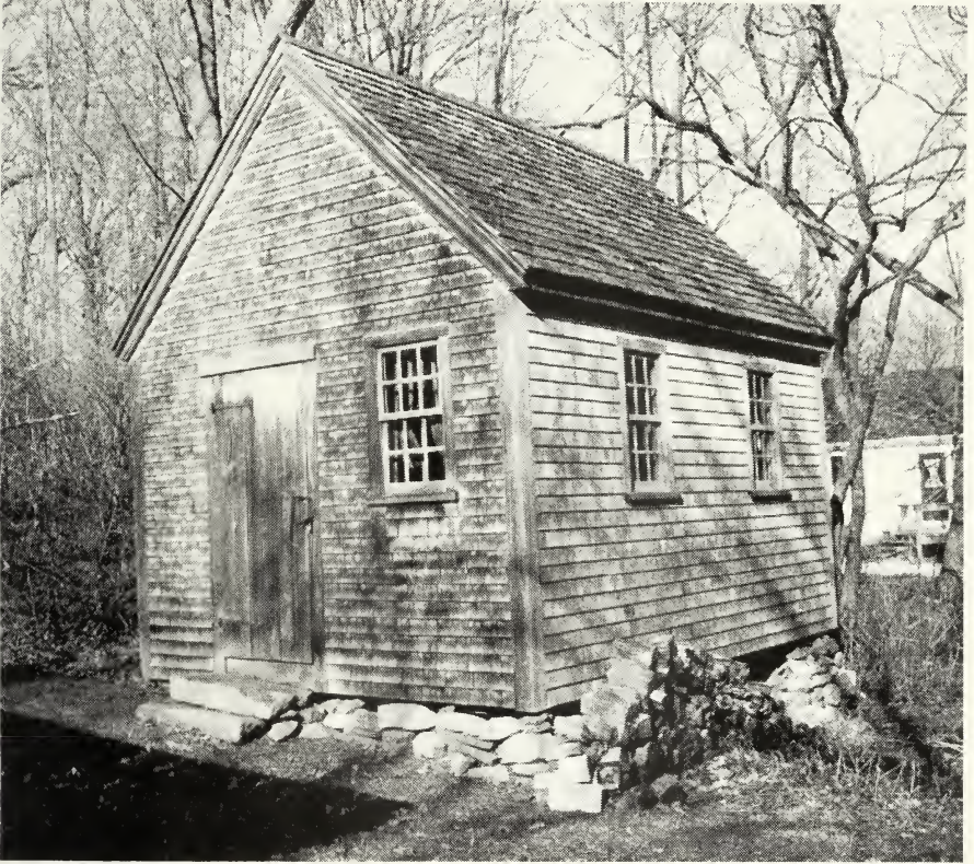
The maintenance building
